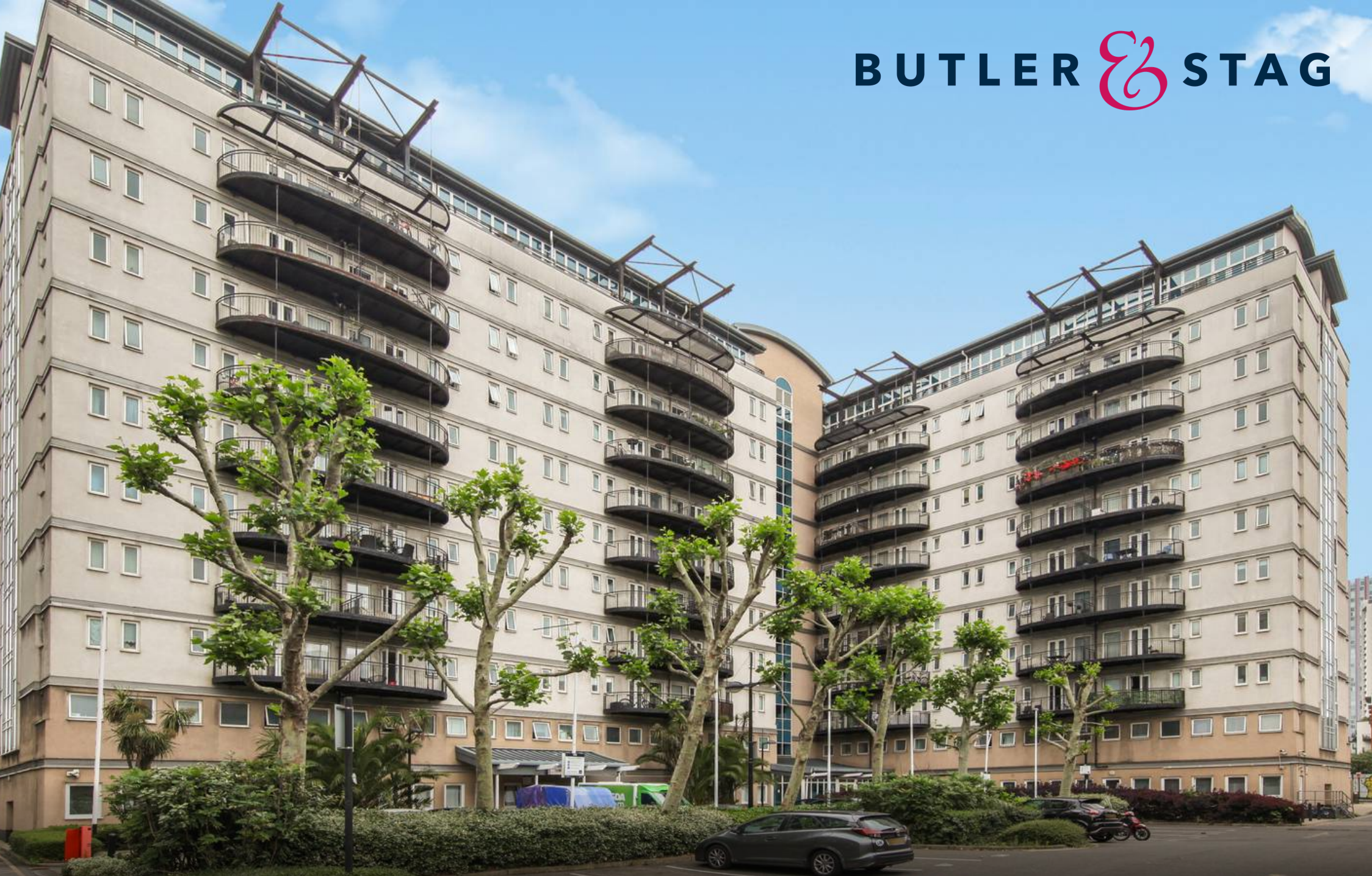
Central House, Stratford, E15 Stratford
